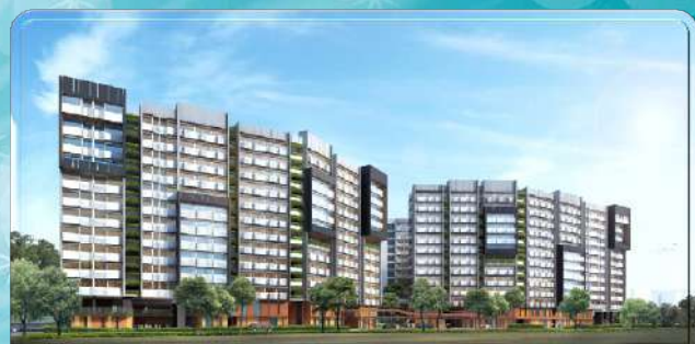
New 1 Block of 11-Sty & 3 Blocks of 13-Sty NTU Student Hostel with MSCP & Ancillary Facilities at Nanyang Crescent (Prefabricated Prefinished Volumetric Construction)
